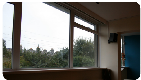
New double glazed windows to replace broken ones in backroom
