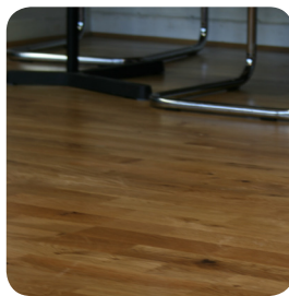
New flooring in office & backroom
